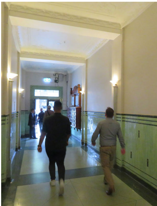
Figure 7 – View of entrance foyer at 94 Oxford Street showing tiled dado terrazzo floors pressed metal ceilings and Inter War lighting.
