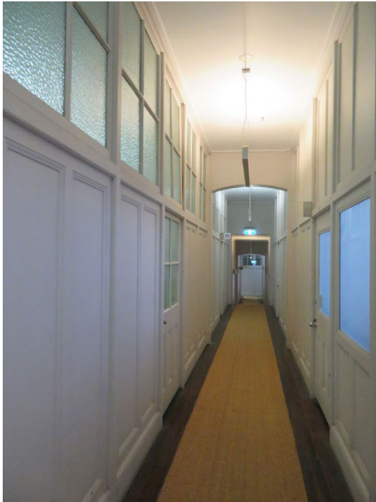
Figure 9 – View of typical corridor in upper floor of building.
