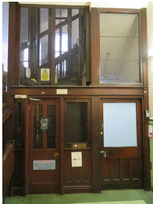
Figure 8 – View of lift and staircase at 94 Oxford Street.
