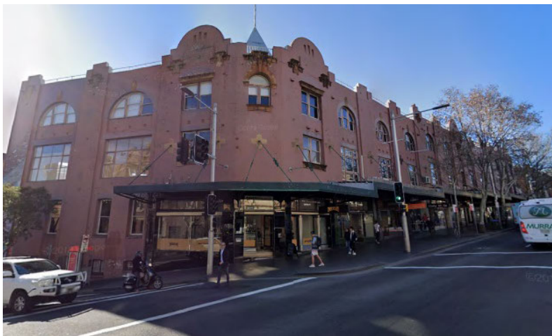
Figure 3 - Exterior view of group 2 building at 82-106 Oxford Street showing the Oxford and Crown Street facades. Source: Google Streetview
