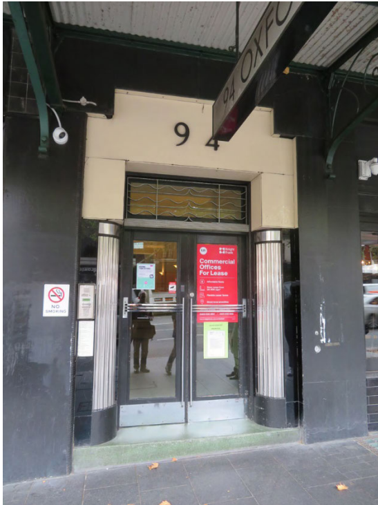
Figure 5 – View of entrance to 94 Oxford Street.
