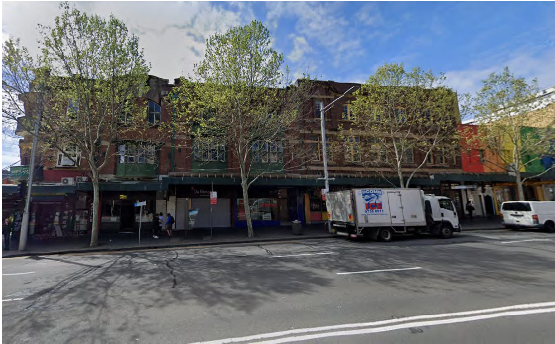
Figure 13 – View of Group 3 buildings (Source: Google Streetview).
