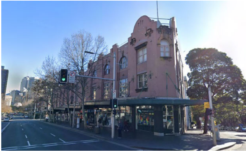
Figure 4 - Exterior view of group 2 building at 82-106 Oxford Street showing the building façade at the corner of Oxford and Palmer Street. Source: Google Streetview
